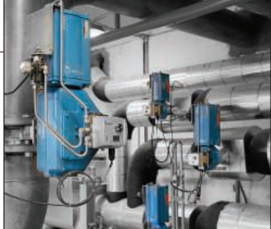
FIGURE 1. Control valves are vital in a variety of industrial applications. Proper design and sizing lead to proper selection, and, ultimately, optimal installation and performance
